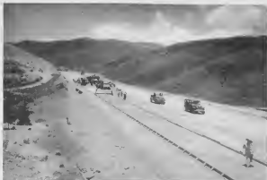
The new highway is 17 kilometers from Catia to Parieta. It's two lanes, each 7.30 meters wide, are separated by an island 1.30 meters wide.
